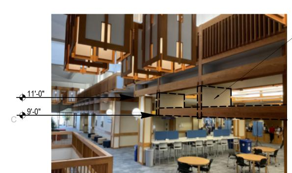
DEMO VALANCE BELOW @9'-0" AS INDICATED ON DEMO RCP, RE.: AD702. PATCH AND REPAIR AS
