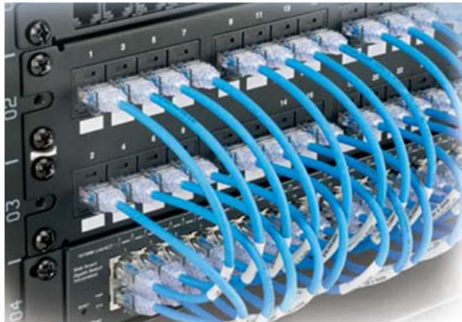
Example of one-to-one switch patching
