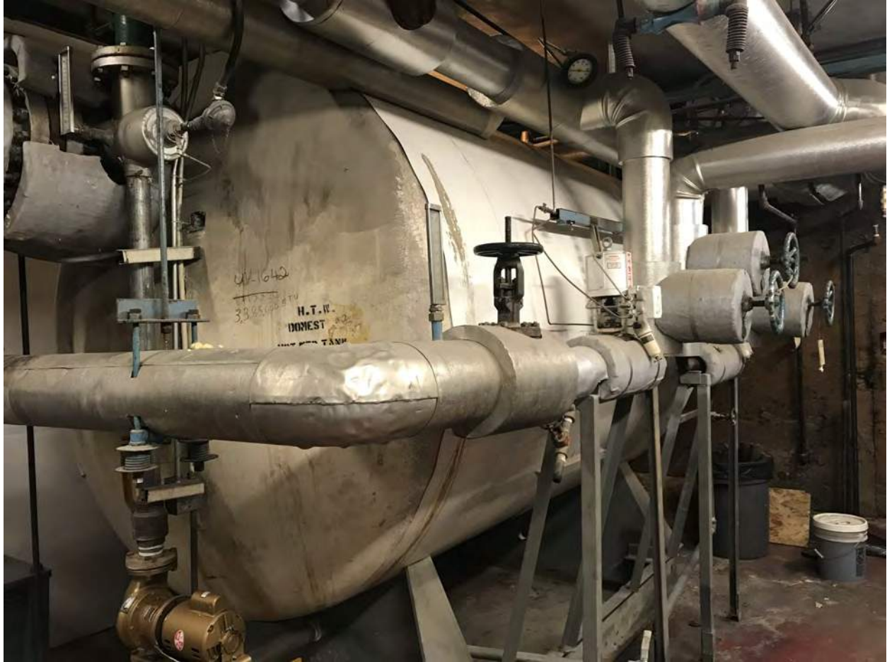
ACM Tank Insulation - Tank 2 by entry - Samples RBB-121820-1 to 3
