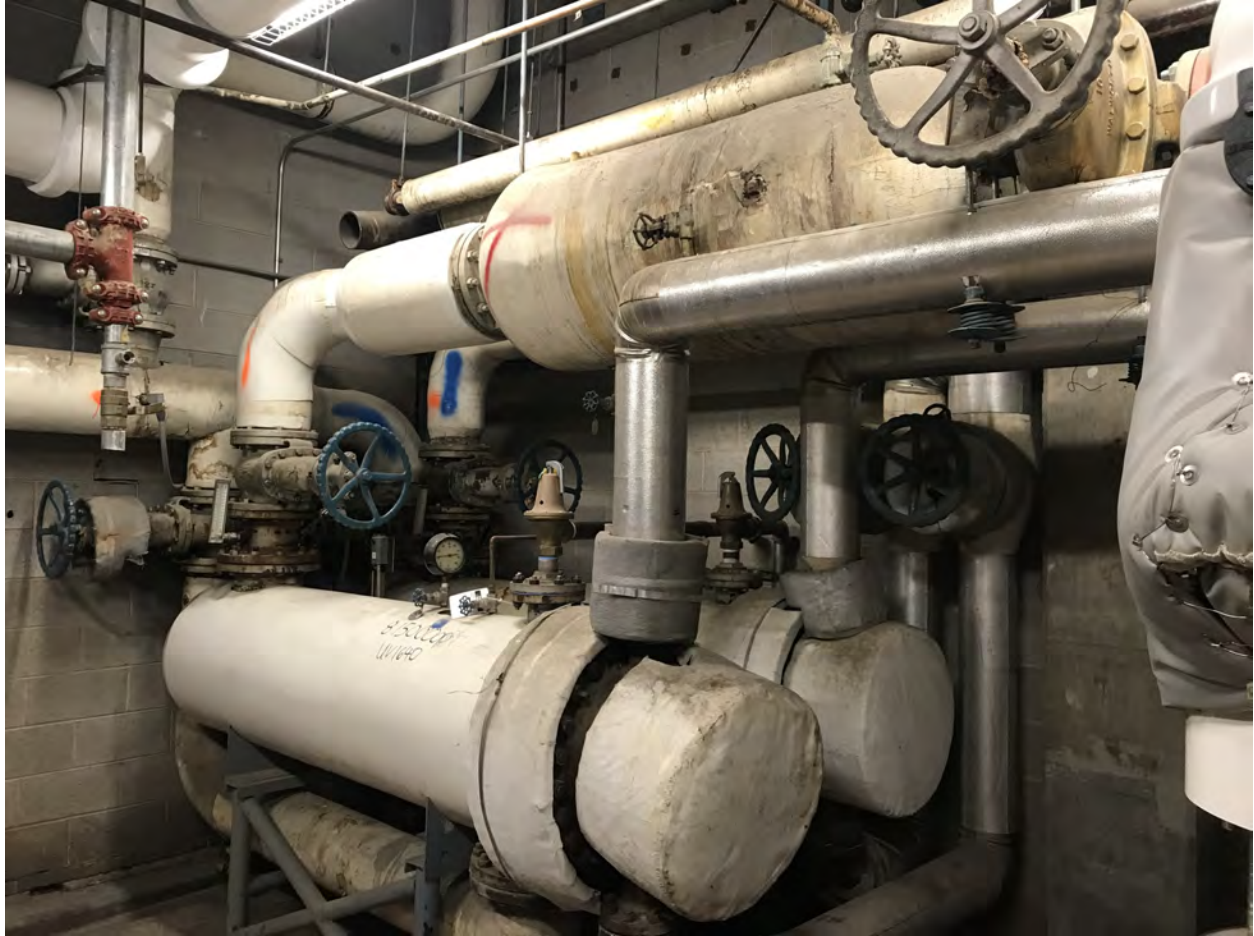
ACM Tank Insulation - Expansion Tanks RBB-121820-14 to 15
