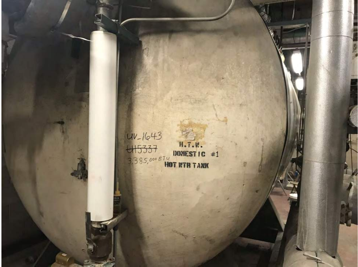
ACM Tank Insulation Tank 1 - RBB-121820-8 to 9
