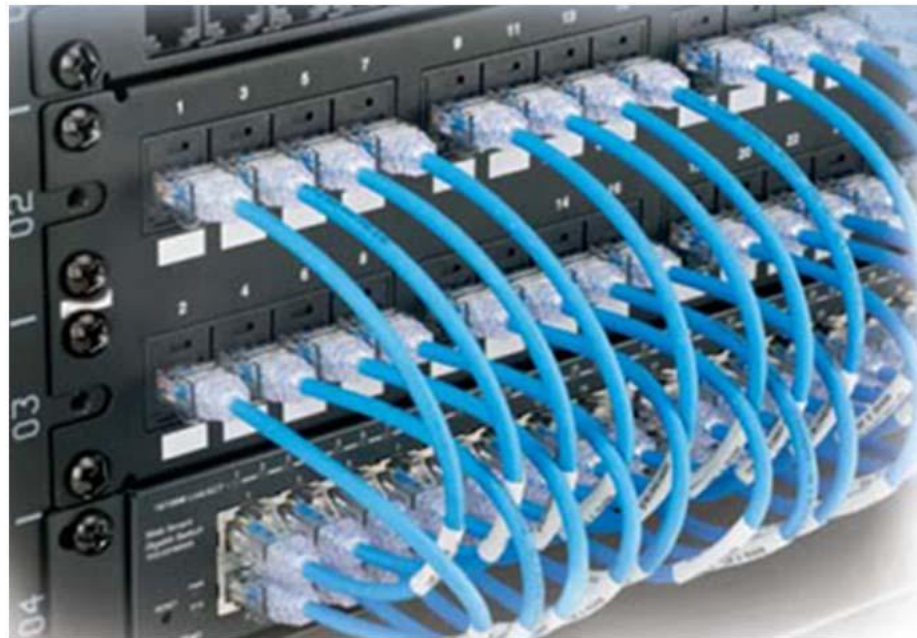
Example of one-to-one switch patching
